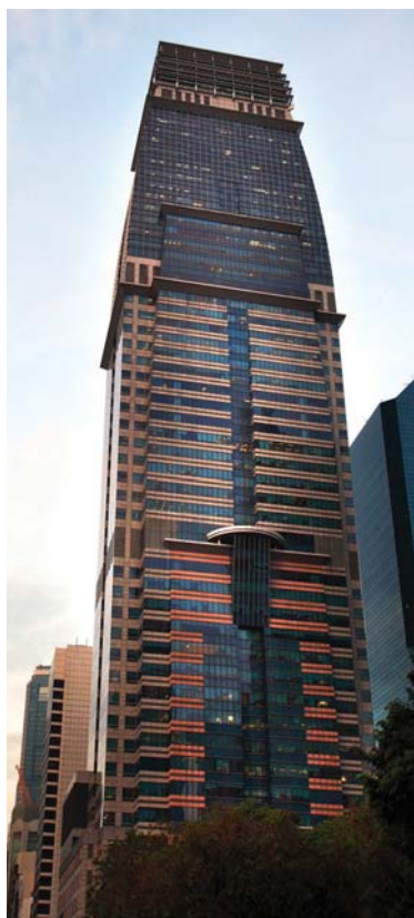
Even though the 52-storey Capital Tower was completed in 2000, it is still valid today, says Lai
