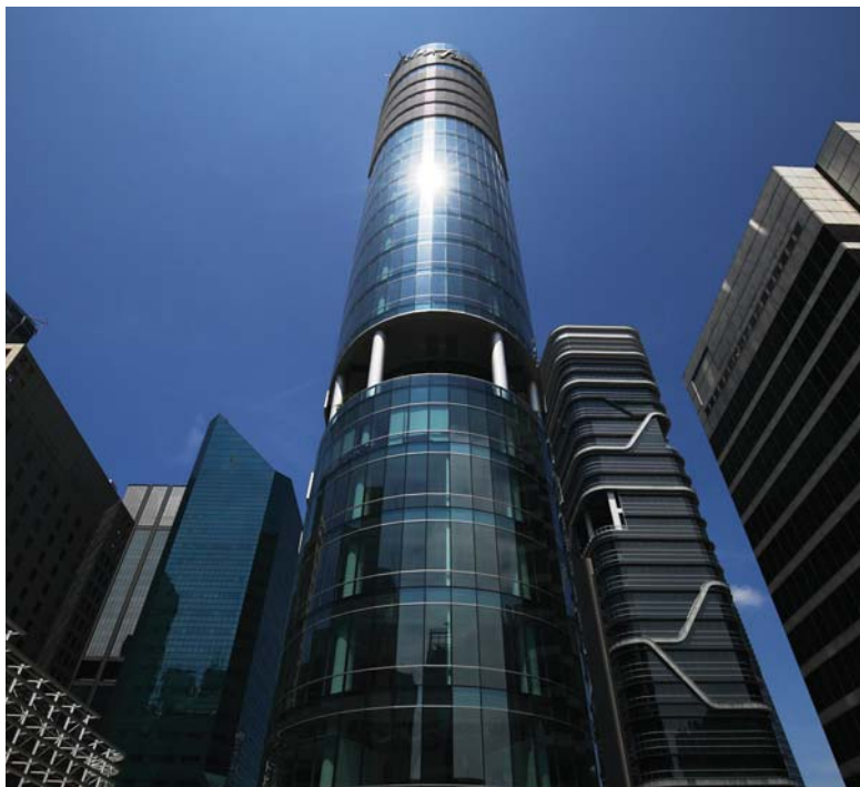
The 32-storey, cylindrical Oxley Tower was completed at the end of last year
