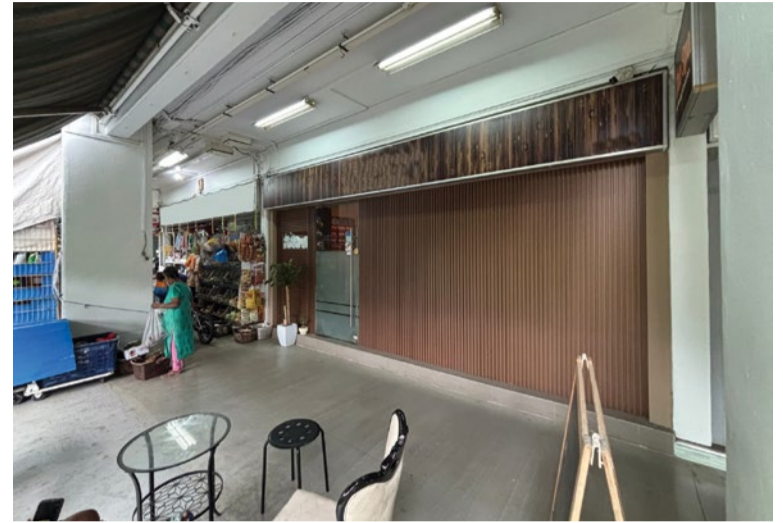
The two-storey shophouse has a floor area of 1,668 sq ft
