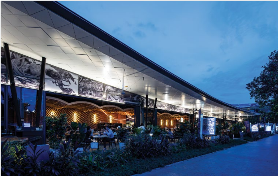
Greenwood Fish Market, an anchor tenant at Quayside Isle, occupies a 7,000 sq ft area with 220 seating capacity at the single-storey block
