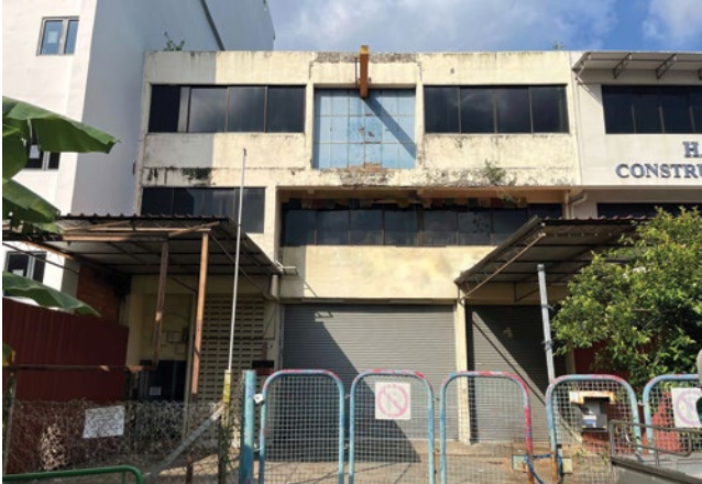
The three-storey terraced factory is situated within Sindo Industrial Estate
